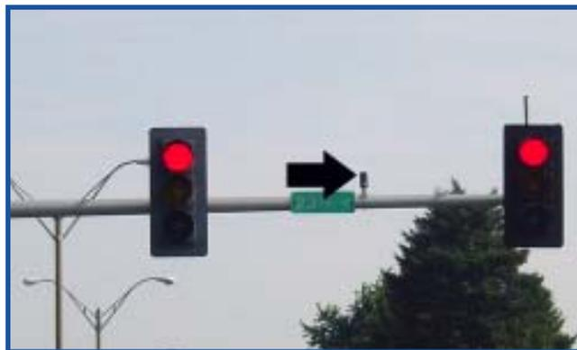
The black arrow is pointing to the Opticom device at an intersection.
