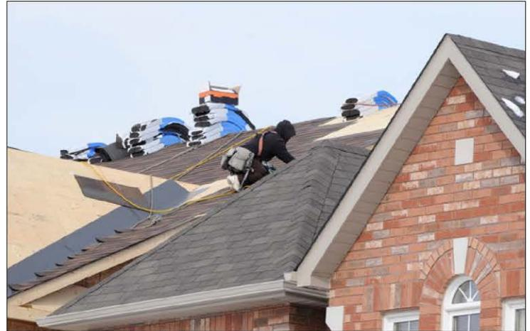
applying the new one. The second would be to lay new shingles over the existing roof. Roofing materials are heavy, so the code only allows one layer of roofing material to be re-roofed over.
