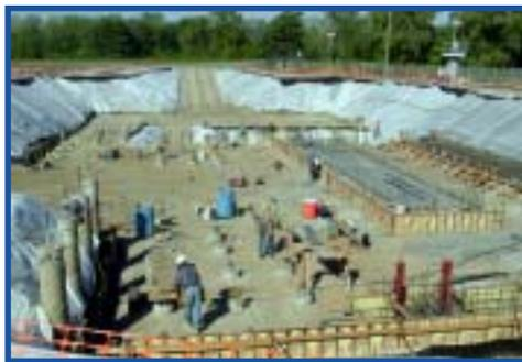
**This new 370,000 gallon clearwell and high service pumping station is being financed with revenue generated by the rate increase. The project, at the Courtney Bend Water Treatment Plant, also includes a 2.5 million gallon storage reservoir directly behind this clearwell.**
